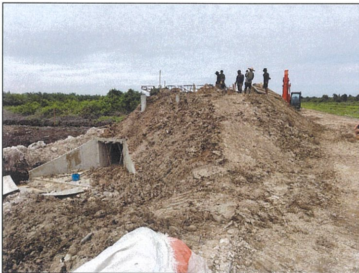
Figure 13. This photo illustrates the ongoing construction of the water pump station intended to house the sludge pump.
