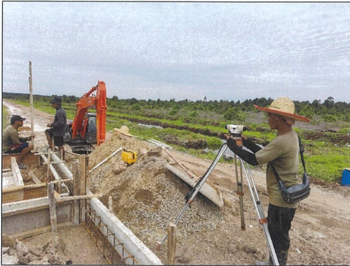
Figure 12. A dumpy level is used to verify the horizontal levels.
